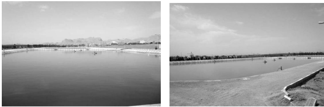
Fig1. Urban wastewater treatment plant with aeration lagoon method from two sides
