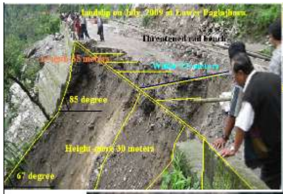
Plate5. Road side failure at Paglajhora (2009) Plate6. A complete distruction in paglajhora(2011)
