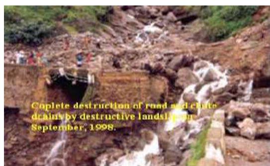
Plate1. Destructive failure in Paglajhor Sinking Zone (1998),
