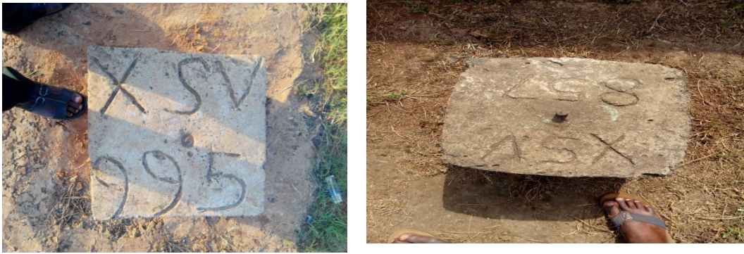
Fig1. Two of the first order federal DGPS controls situated at Adazi-Nnukwu, Aniocha Local Government Area with inscription XVS 995 and Ekwulobia, Aguata Local Government Area with inscription XVS 857, both in Anambra State
