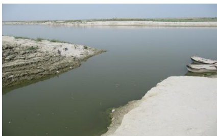
Photo13. River water backflow into Dabka Drain at Confluence point
