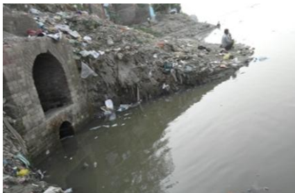
Photo7. Confluence of Parmath drain having dry
