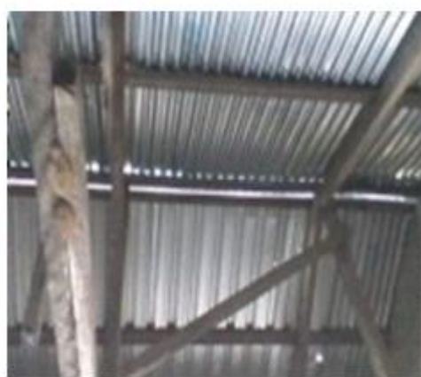
Partially de-roofed staffroom in use
