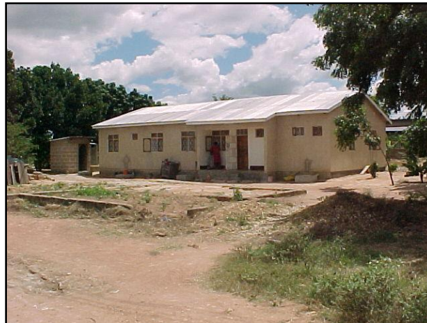
Fig1. A house constructed through cooperative efforts in Dodoma, Tanzania.
