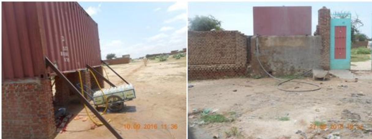
Board1. Water drilling at Amrié (Dombor, September 2016)
