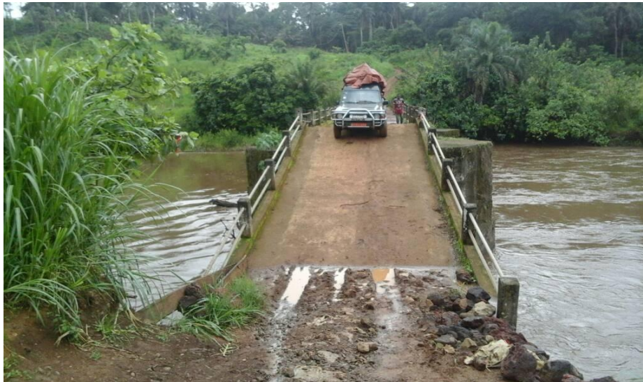
Picture III: the Mugu Bridge constructed by BEDECA in 1998
