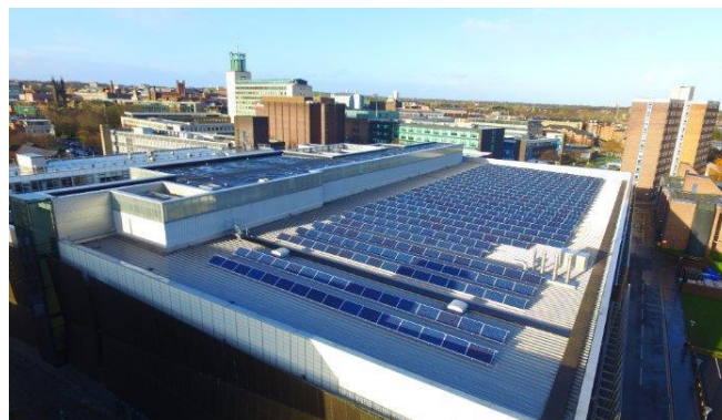
Fig3. Solar Panels and Rainwater Harvesting Systems
