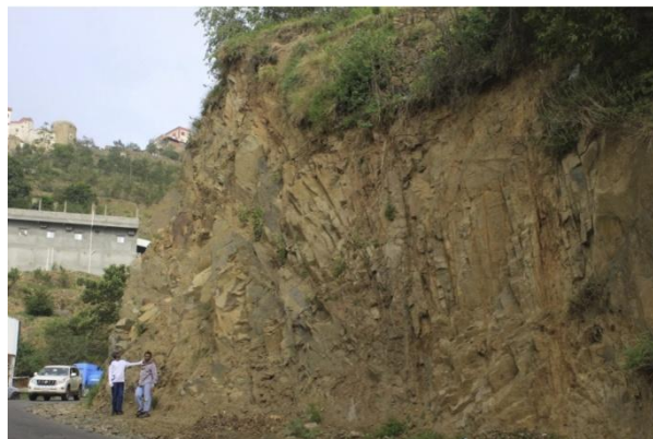
Fig5. Potential for flexural toppling failure [26]
