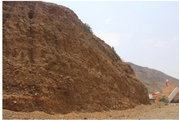
Fig3. Example of non-structurally controlled failure due to highly weathering [26]
