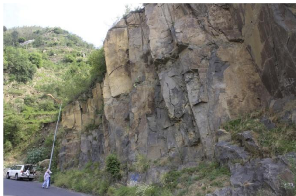
Fig6. Potential for block toppling failure [26]
