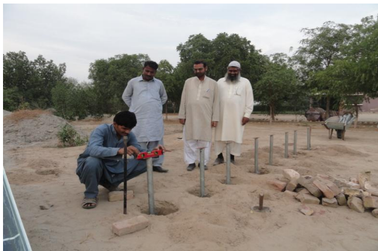
Zero level of poles installation for desalination mounted on pole
